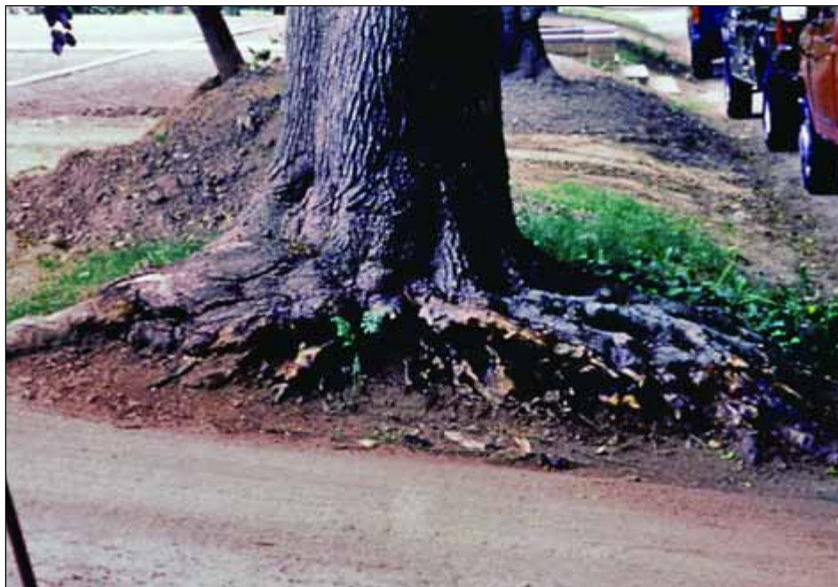
Root damage to a Norway maple; such damage is often covered by new plantings or turf and might not be immediately visible.
